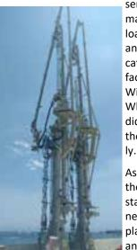
sembly and erection of the five (5) marine loading arms. These marine loading arms, which supply both JP5 and DFM Fuel to the ships were fabricated at Emco-Wheaton's Germany facility and shipped in 15 containers. With the oversite of an Emco-Wheaton representative, our crews did a tremendous job assembling these large pieces of equipment safe-ly.
